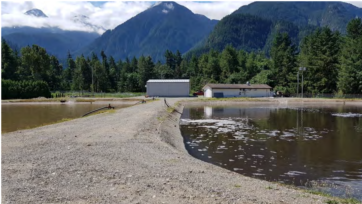
FIGURE 3-3: DISSOLVED AIR FLOTATION BUILDING, BLOWER BUILDING AND LAGOONS
