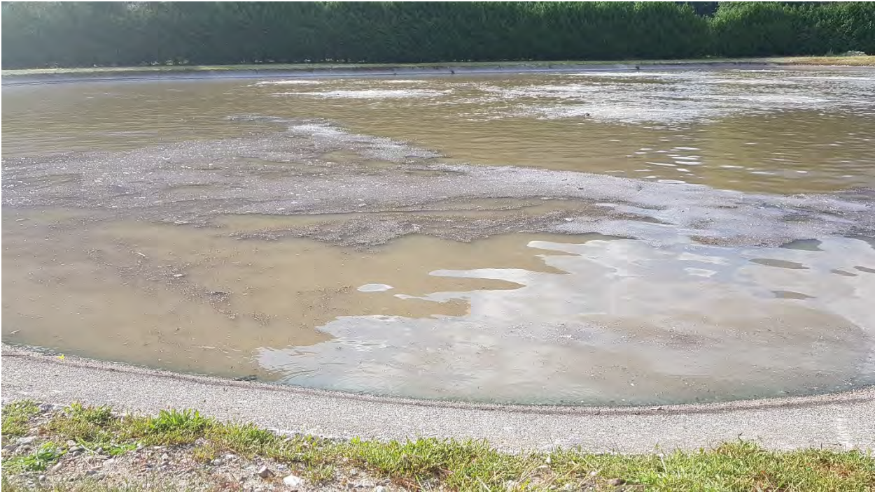
FIGURE 3-6: EXAMPLE OF AN AERATION DIFFUSER FOULED WITH RAG
