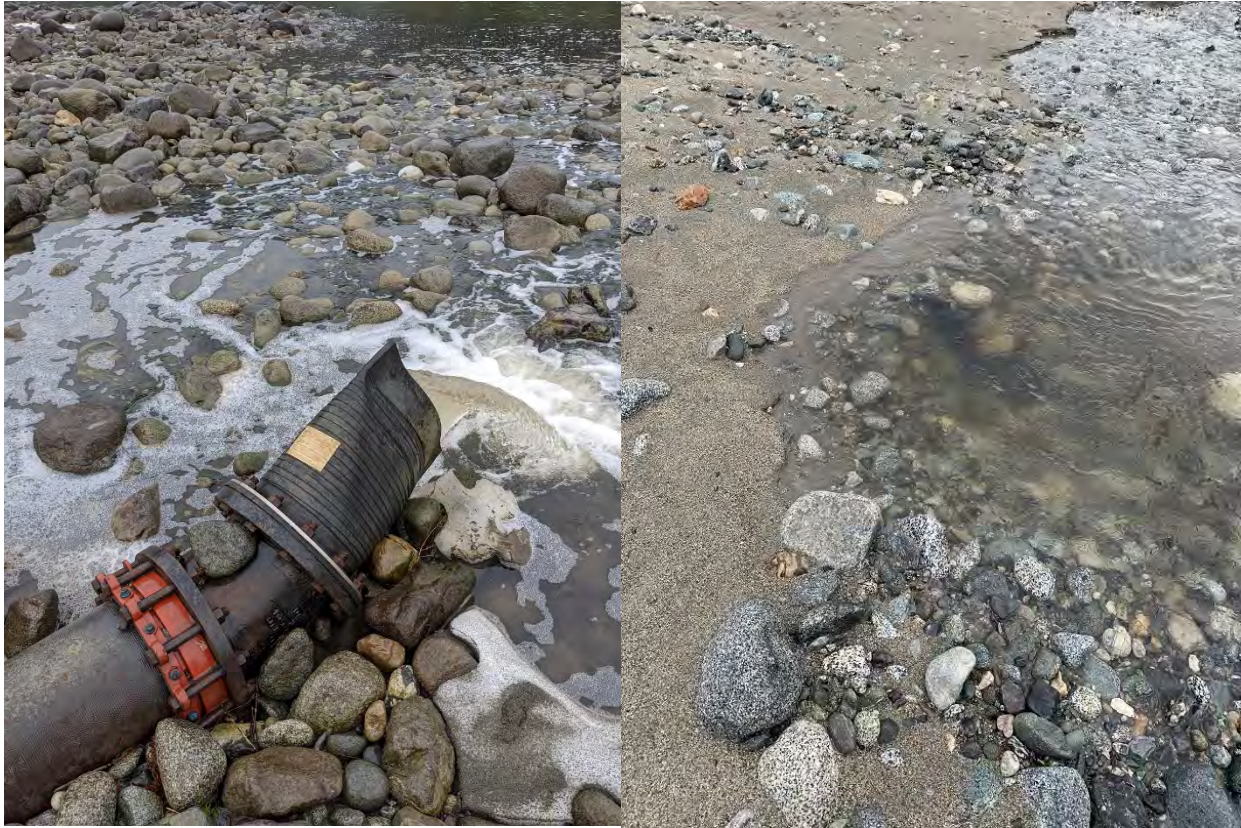
FIGURE 3-9: TEMPORARY OUTFALL JANUARY 23, 2020 (LEFT) AND FEB 13, 2020 (RIGHT)
