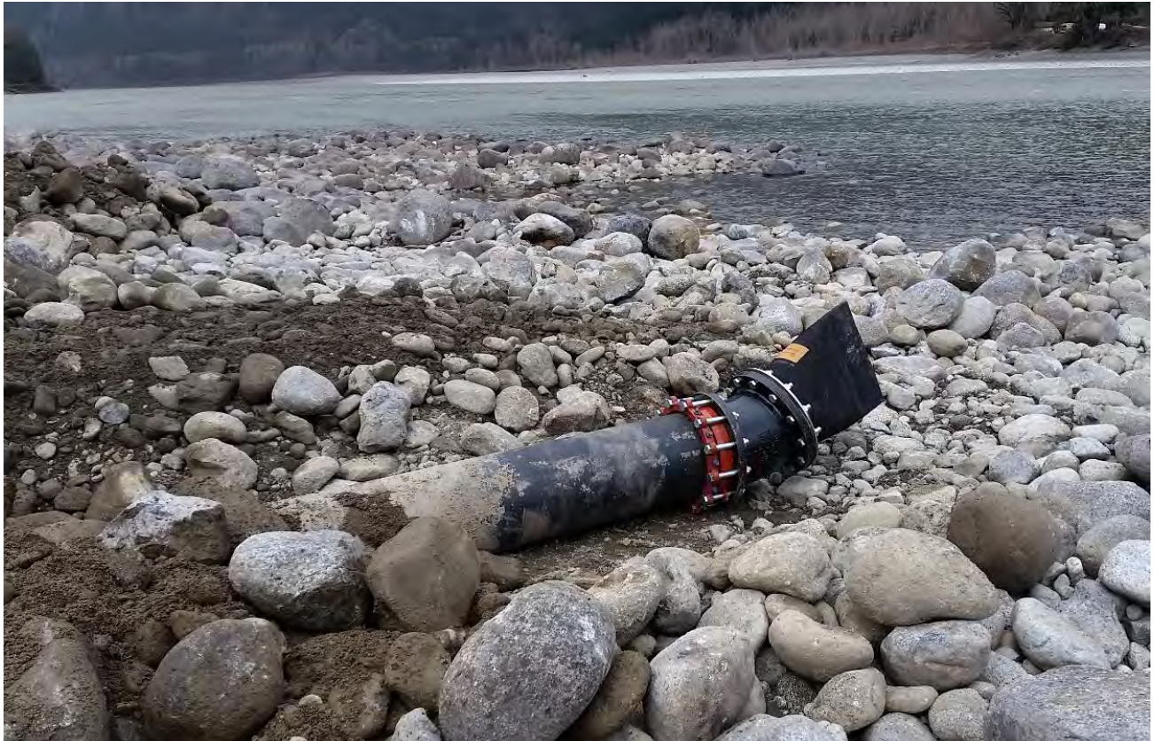
FIGURE 3-8: TEMPORARY OUTFALL AT TIME OF CONSTRUCTION
