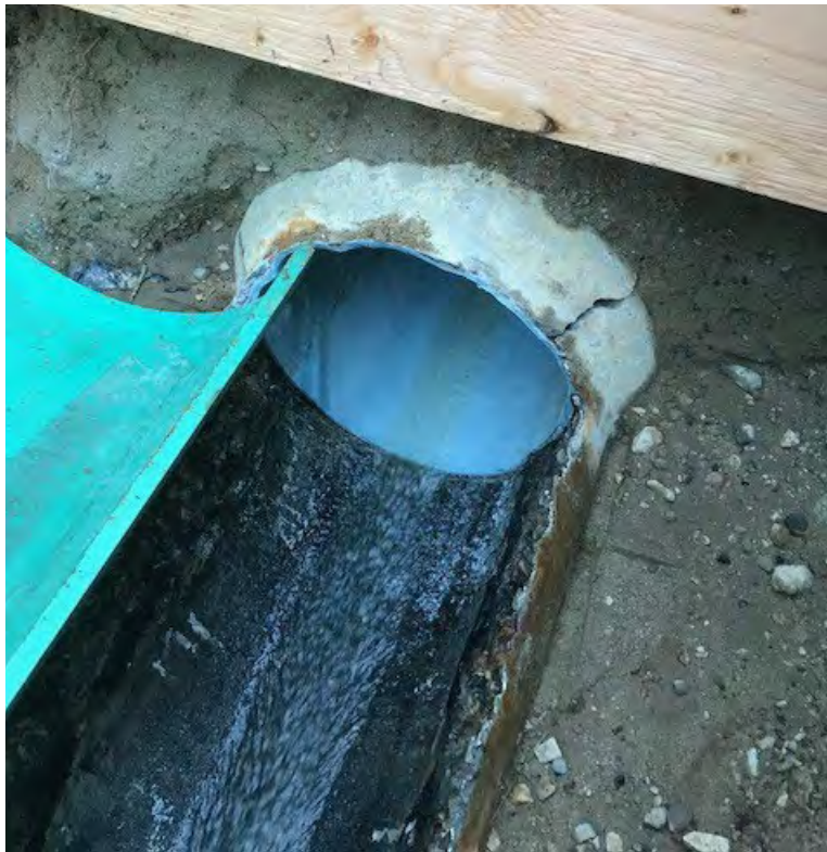
FIGURE 3-1: FRESHLY LINED FORCEMAIN
