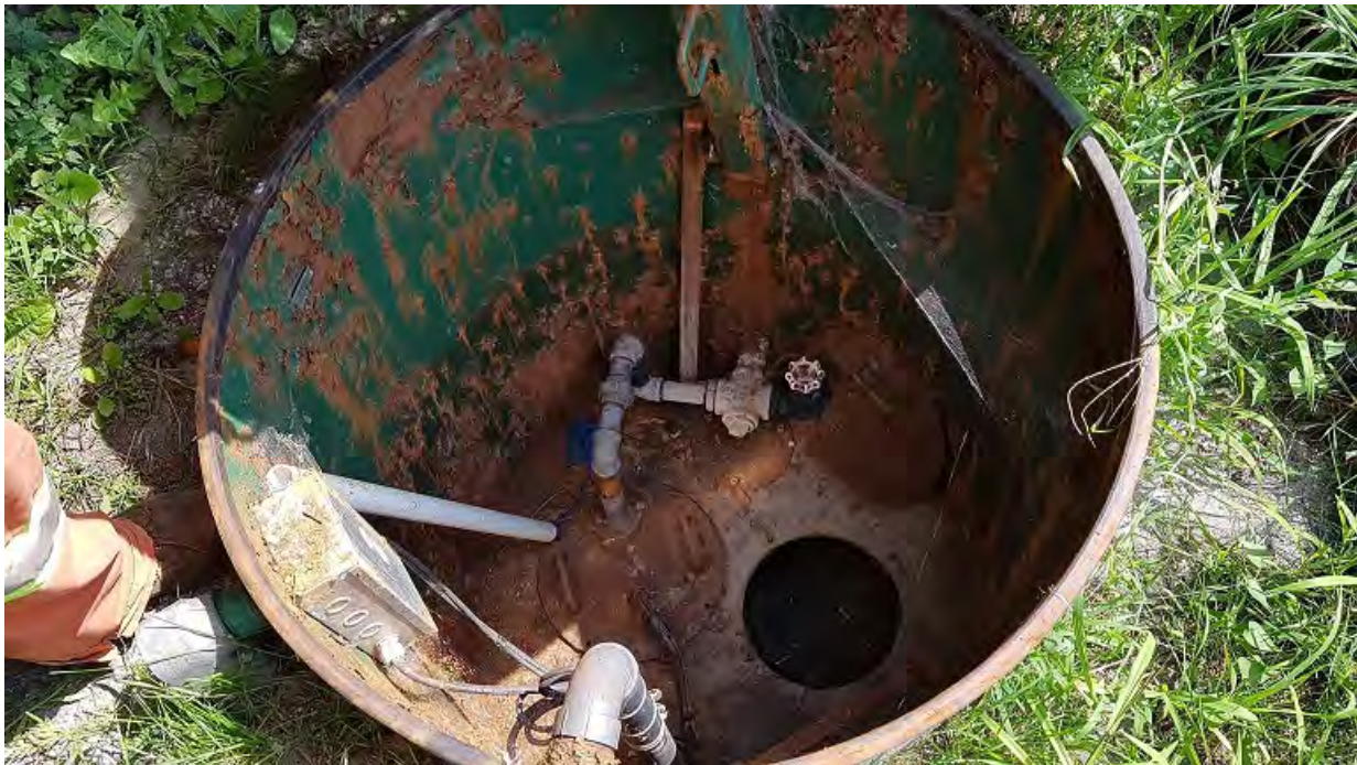
FIGURE 3-2: UNION BAR LIFT STATION
