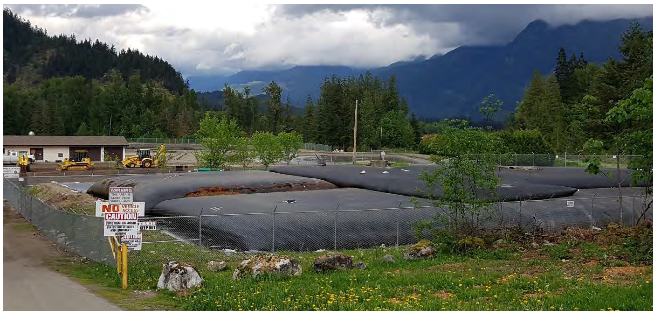
FIGURE 3-7: GEOTUBE BAGS CONTAINING SLUDGE REMOVED IN 2017.
