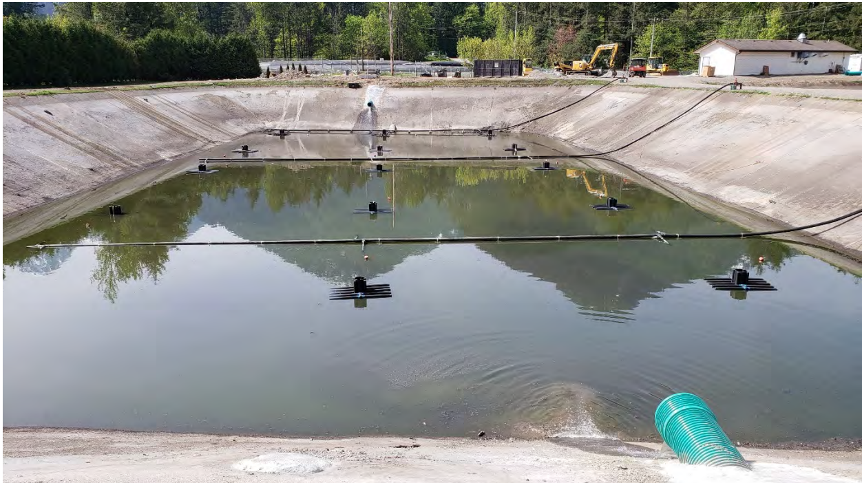
FIGURE 2-6: INSTALLATION OF NEW AERATION SYSTEM INTO CELL #1 (MAY 2018)
