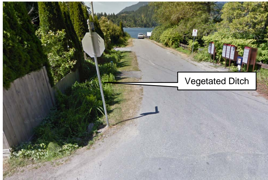
FIGURE 4-5: ENCOURAGEMENT OF VEGETATION IN DRAINAGE DITCHES REDUCES VOLUME AND FLOW CAPACITY
