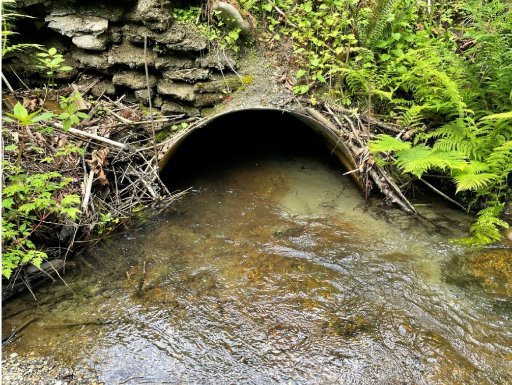
FIGURE 4-4: EXAMPLE OF CULVERT REQUIRING MAINTENANCE TO INCREASE CAPACITY
